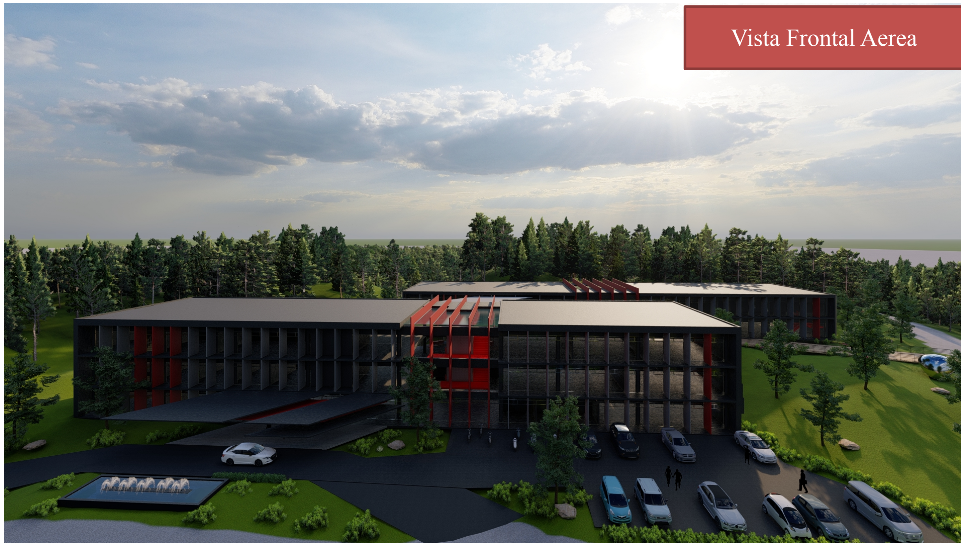
Vista No.1 Exterior Frontal Aerea
