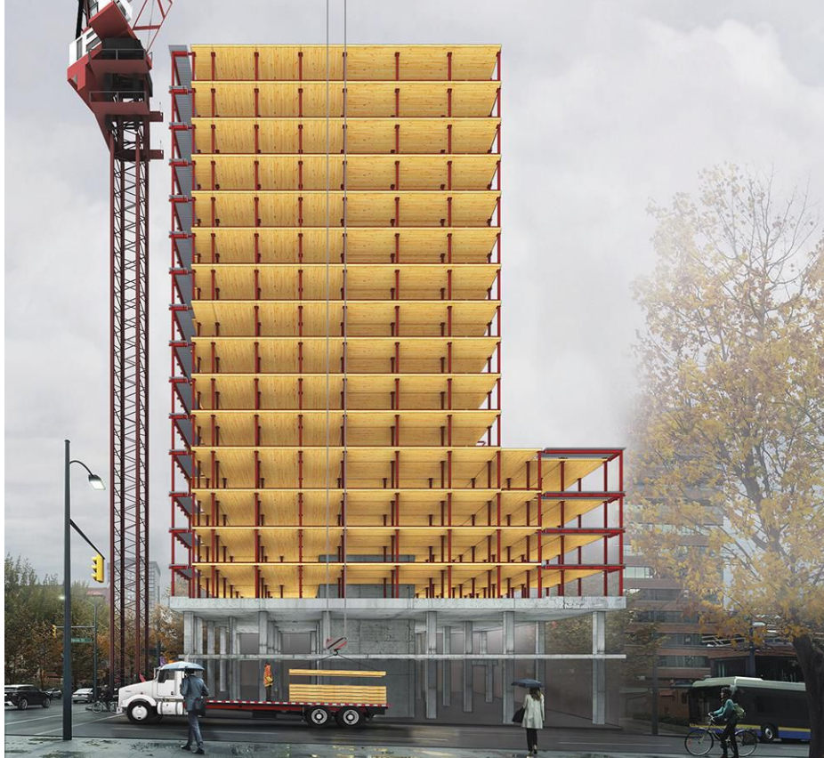
A STRUCTURAL SYSTEM combining CLT slabs and steel columns (above) should speed construction at 981 Davie (opposite), in Vancouver, British Columbia. The building will provide 154 affordable units.
