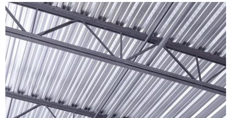
Composite joists and deck
