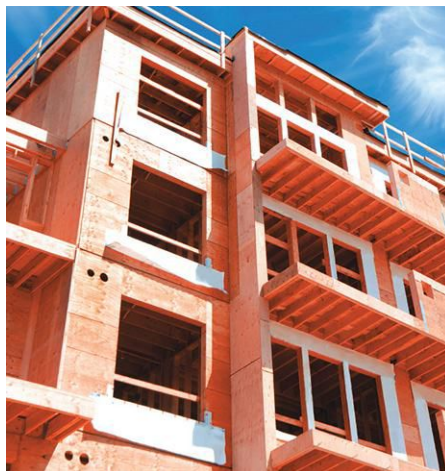
Fire-retardant pressure-treated wood (FRTW) is recognized as a code-acceptable option for framing walls and roofs for many multifamily buildings.
