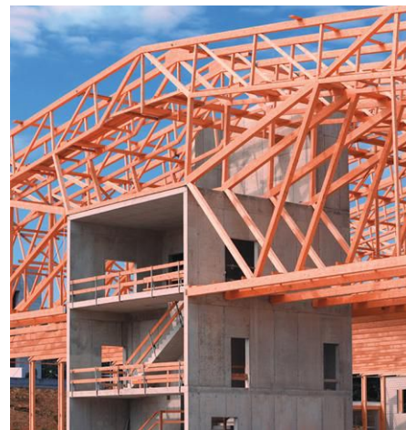
Fire-retardant pressure-treated wood (FRTW) is recognized as a code-acceptable option for framing walls and roofs for many multifamily buildings.
