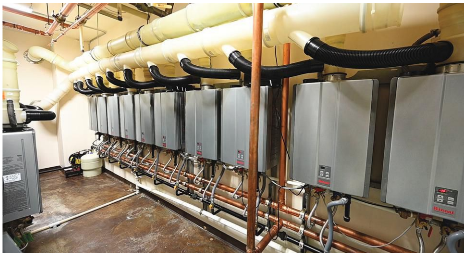
An array of tankless water heaters at Ruby's Inn saves energy and space and provides reliability to keep the establishment running smoothly.
